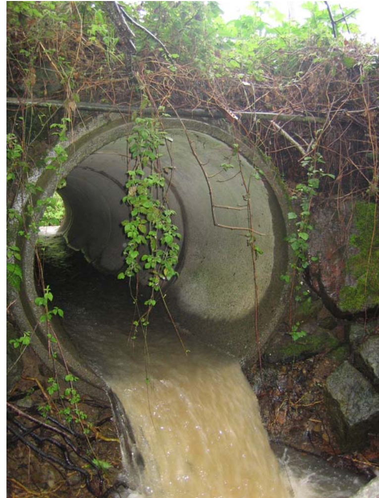
Figure 1. Juvenile coho were found by DFG biologists in the pool just below this barrier, unable to migrate upstream (Sept. 2006).
