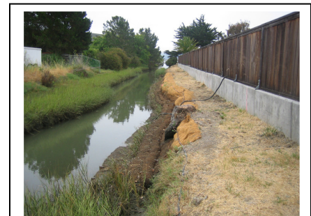
Post-Coir Log Installation
