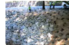
Bank stabilization project at Creek Road Bridge
