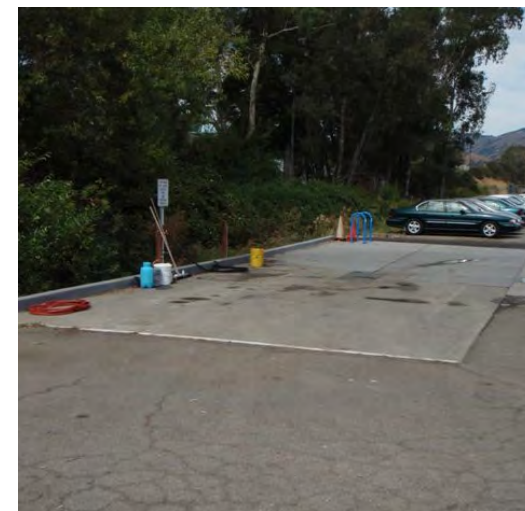
The County’s Corporation Yard wash pad was upgraded to ensure all washwater drains to the sanitary sewer.
