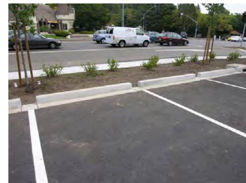
Bioretention featured in a bank parking lot in Corte Madera
