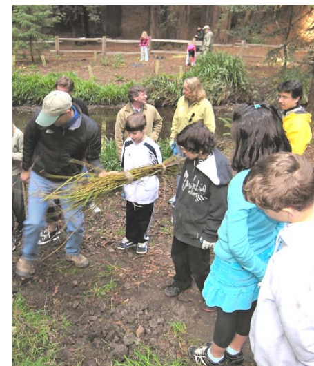
Showing students how to install fascines
