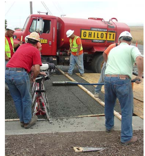
Pervious concrete installation (CSWST2)
