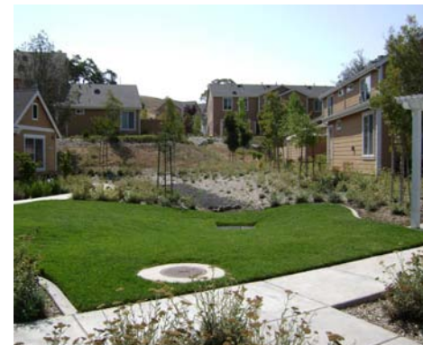
Low Impact Development features in Novato’s Meadow Park subdivision (photo by CSWST2)
